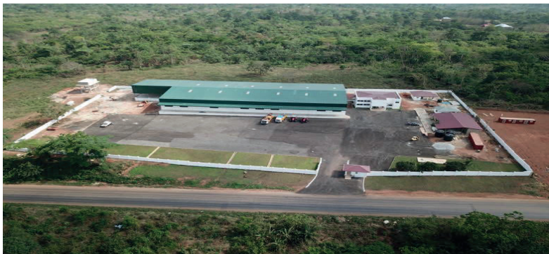
Tomato Processing Factory at Domfete, Berekum West under 1D1F
