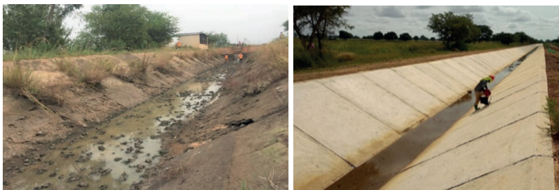
Rehabilitation of Tono Irrigation Project, Navorongo
