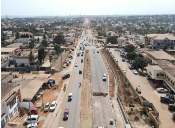
La Beach Road Completion Project
